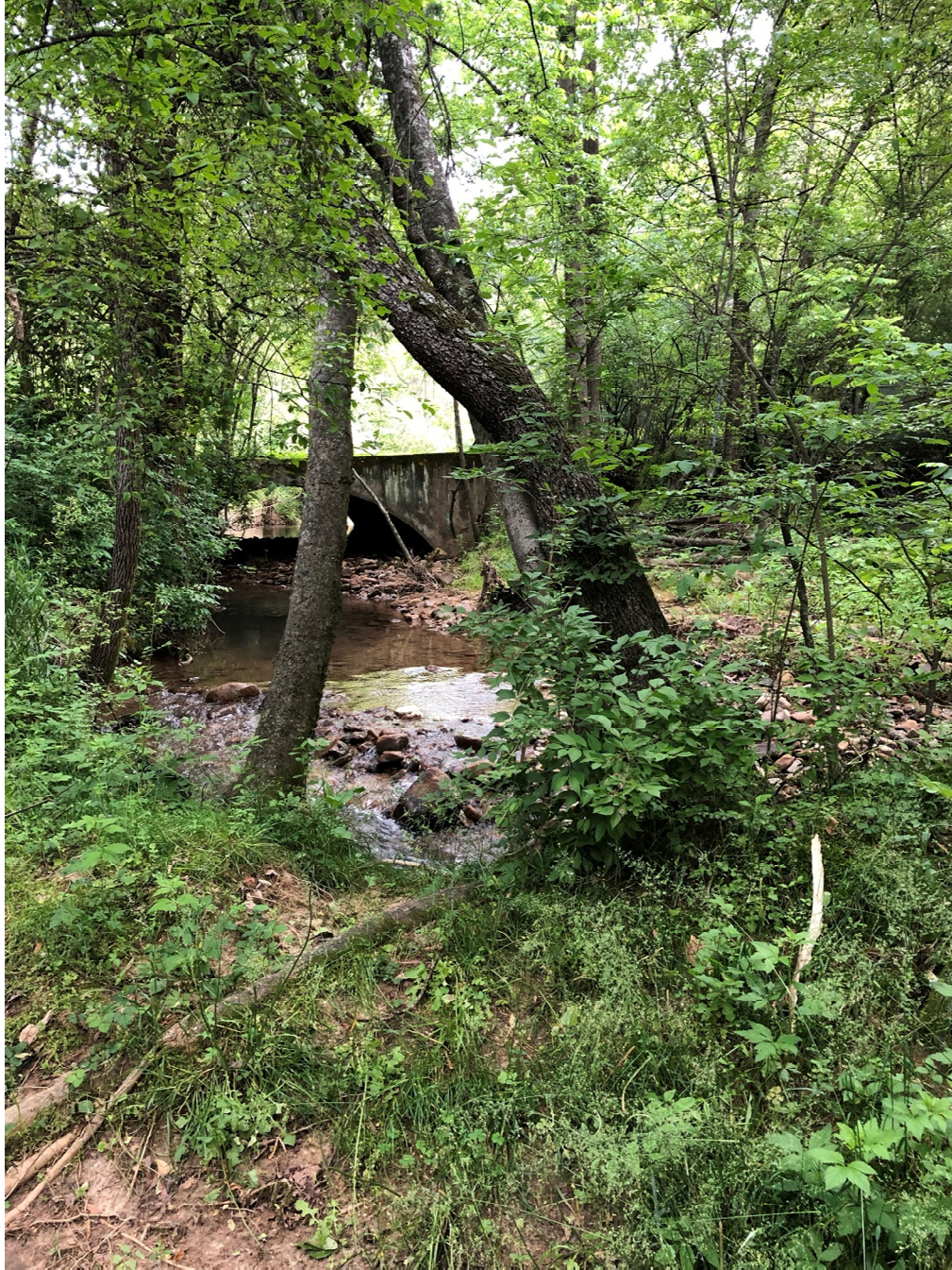
Picture 6: In front of stream bend facing north, where bank will be lowered to approximately 12”
